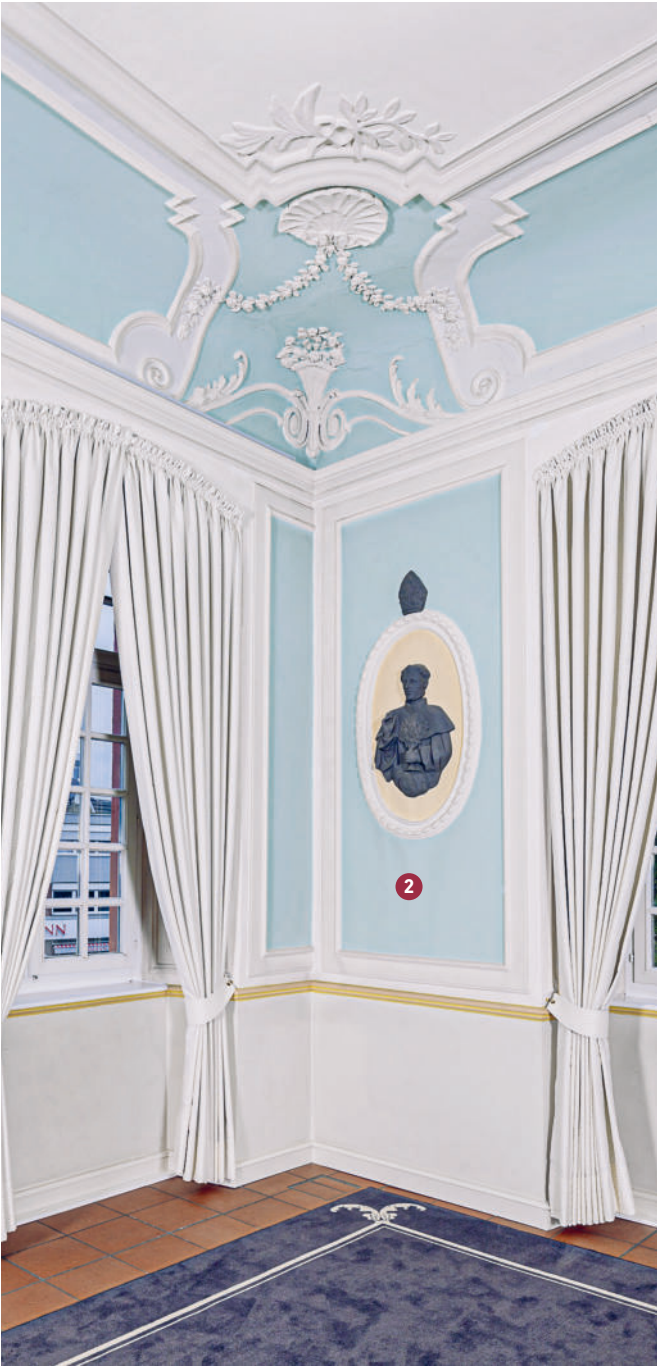
Alongside the ostentatious decoration of the exterior façade, the design of the Abbot's hall seems more akin to the restrained phases of Rococo or Classicism that soon followed the Baroque.
